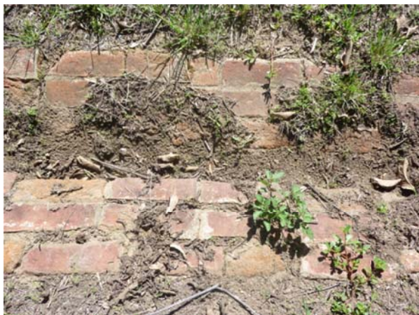
Section of brick drain, Noble Street
