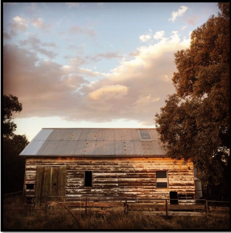
19 th Century shearing shed, repaired & adapted to 21 st Century work shed, Sheans Creek. Image: C. Hammond 2018
