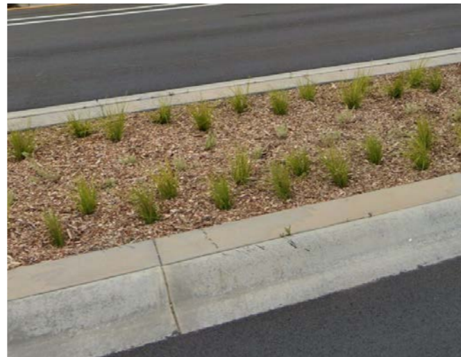
Concrete maintenance edge along median
