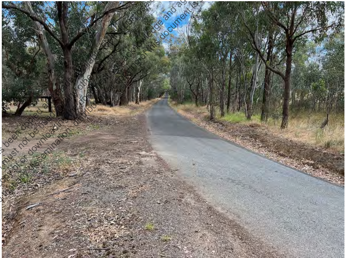
Figure 8 – Seven Creeks Estate Road alongside the eastern boundary
