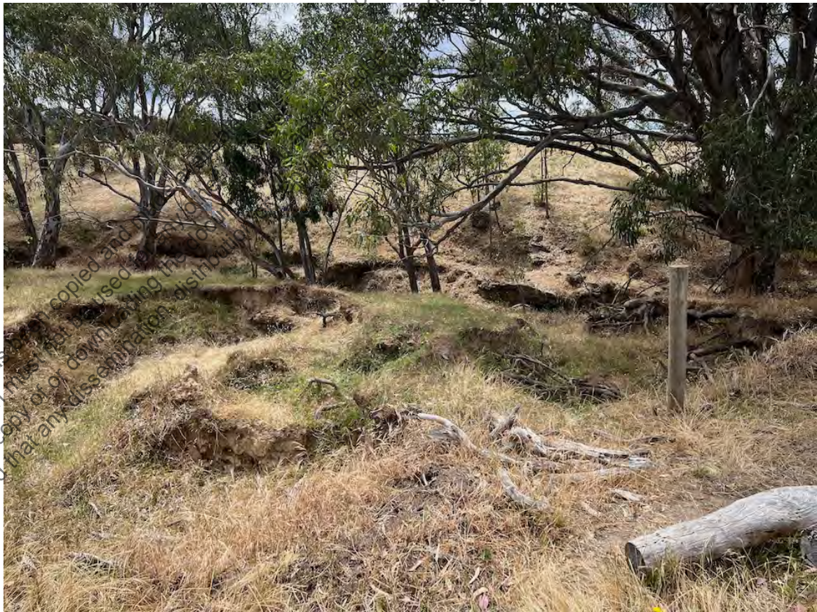
Figure 58 - Gully erosion on the property
