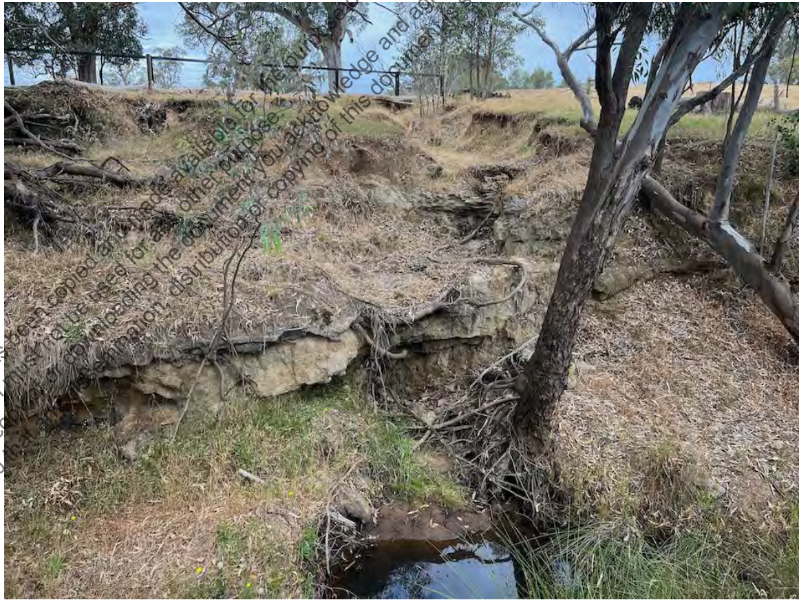
Figure 60 – Erosion where the creeks/gullies meet on Lot 2
