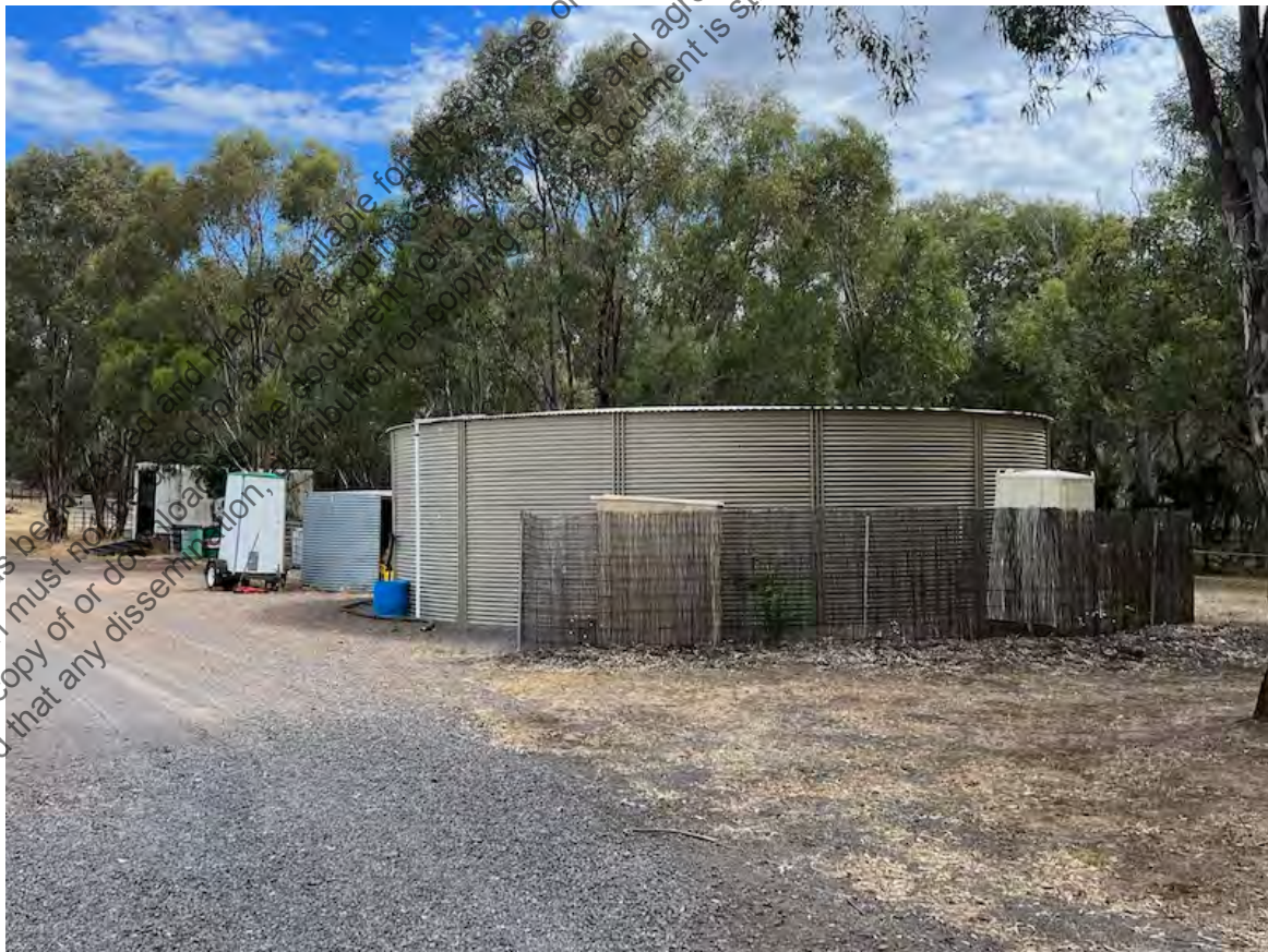
Figure 16 – Water tank on Lot 1
