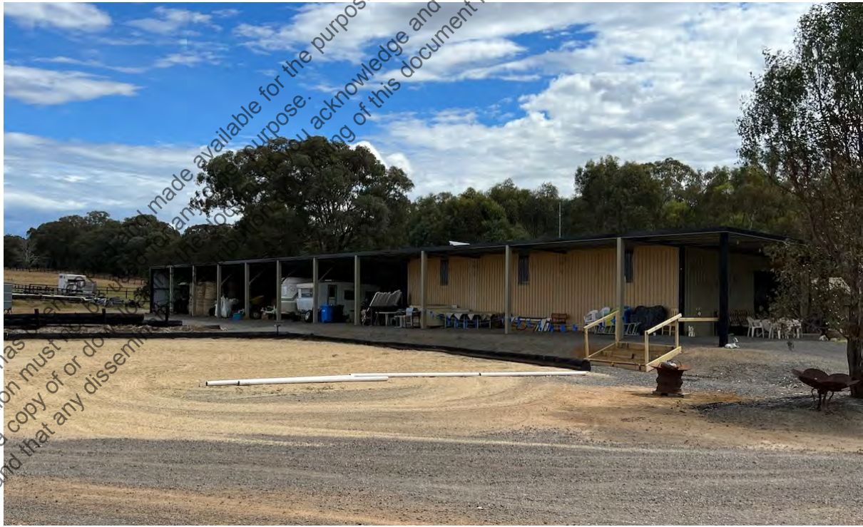
Figure 18 – Stables and storage shedding on Lot 1
