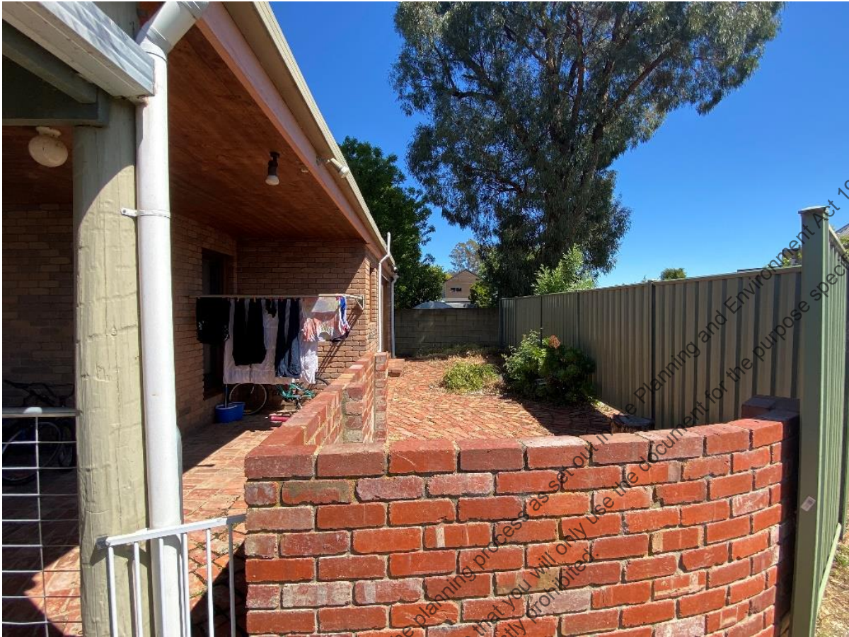
Figure 7 - Existing fencing separating the front dwelling to the rear building (October 2023)
