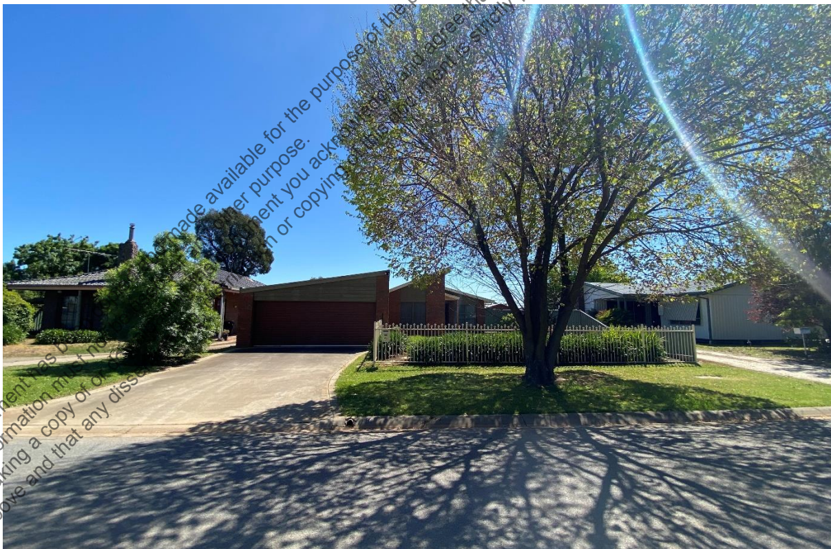
Figure 14 - 28 River Street (adjoining eastern property), with car parking garage within the front setback (October 2023)
