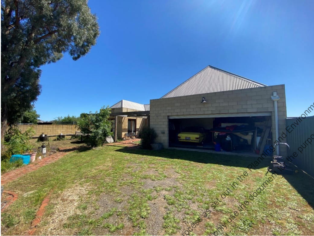
Figure 5 - The existing rear building as seen from the driveway (October 2023)
