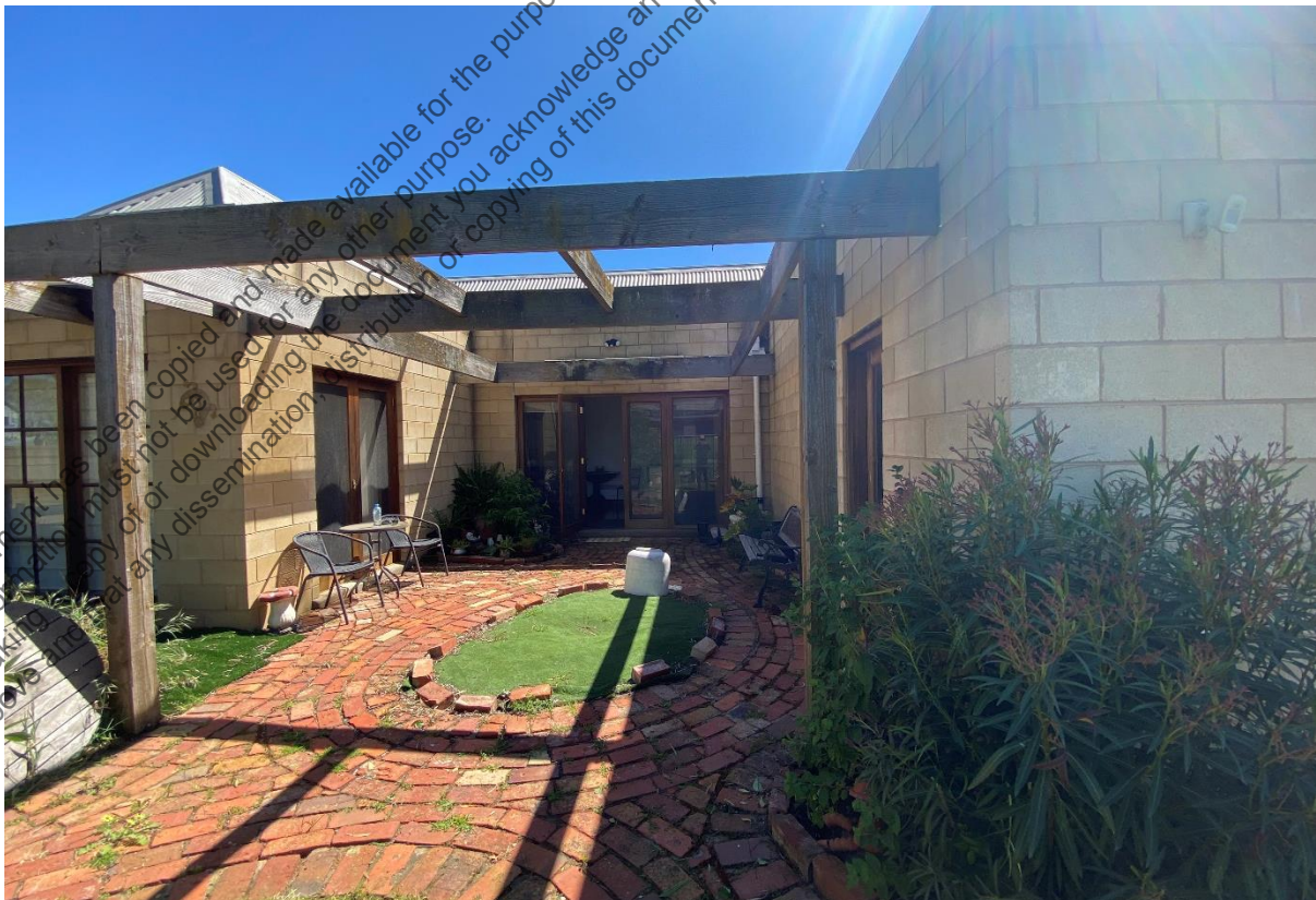
Figure 8 - The front of the existing rear building (October 2023)
