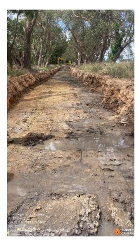
During the execution of the treatments, active springs were encountered in the subgrade of the failed pavements which required treatment as variations to the Contract. The number of sites where this has been encountered has resulted in the cost of the treatments being greater than 10% of the original contract which subsequently requires Council approval.
