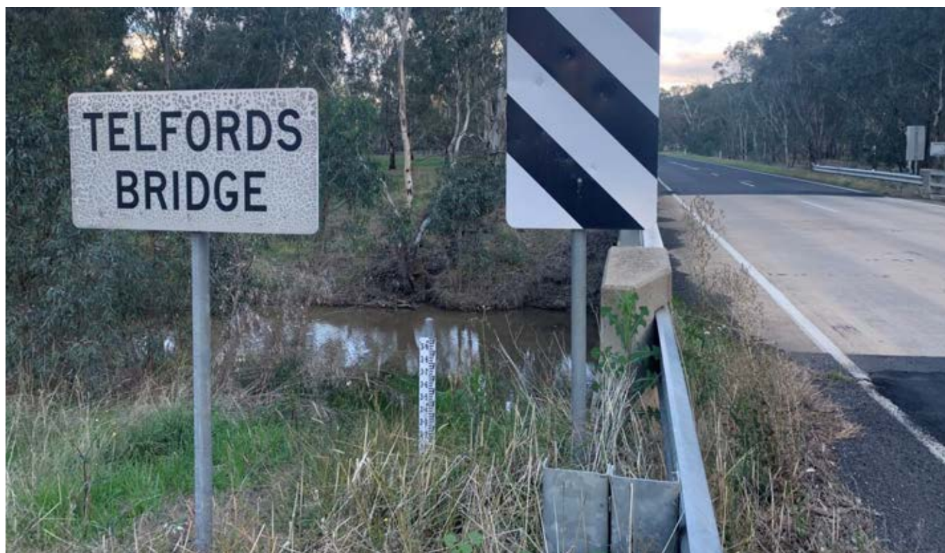
Castle Creek Gauge at Telfords Bridge on Euroa-Mansfield Rd.
