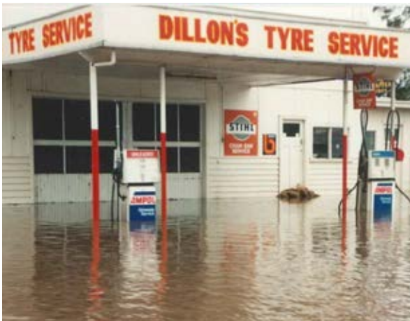
Williams Garage, previously Dillon's Tyre Service during the flood in October 1993. Image from Strathbogie Shire Council.
