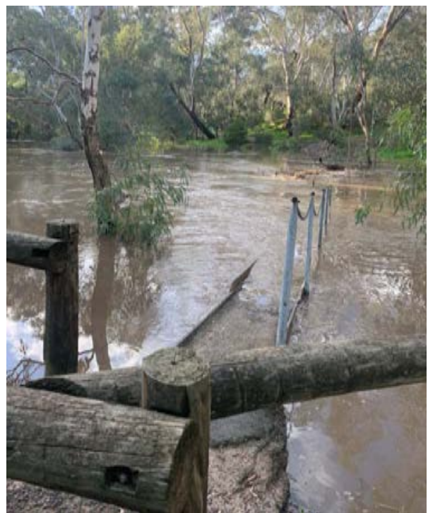
Rockies Bridge downstream of the Seven Creeks Gauge at Euroa during the flood in April 2020.
