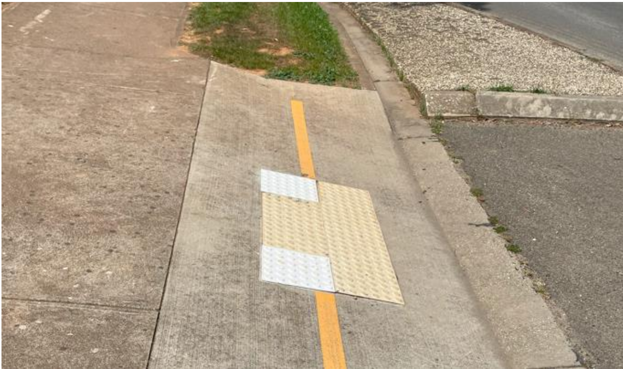
It is recommended that the TGSIs are installed covering the “full width of the path of travel - perpendicular to the direction of travel”. Incorrectly installed TGSIs could lead to vehicle/pedestrian crashes.
