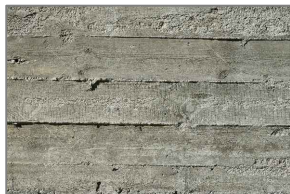
OFF FORM CONCRETE DETAILING
