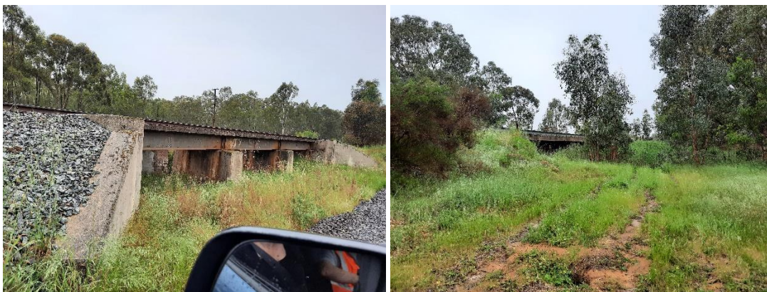
Figure 10. Photo location 1 and 2: Railway crossings representing hydraulic model outlet.
