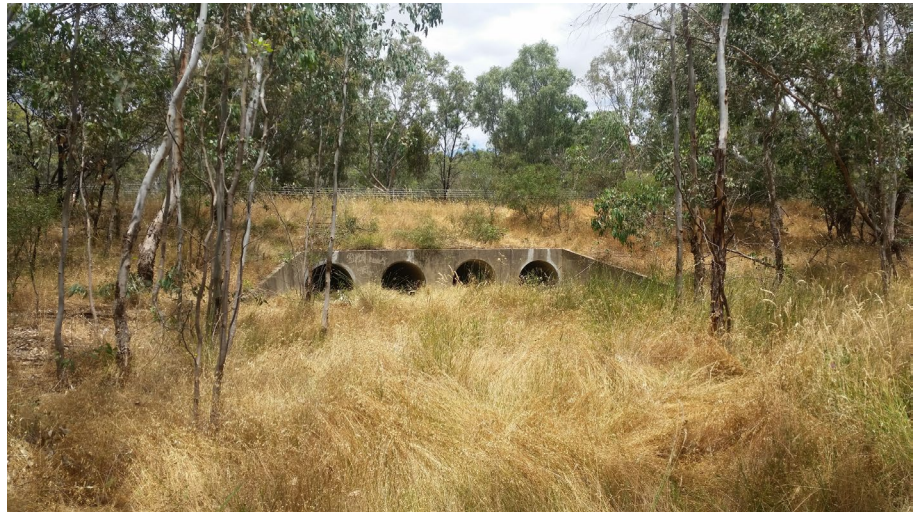
G – Culverts under the Hume Freeway
