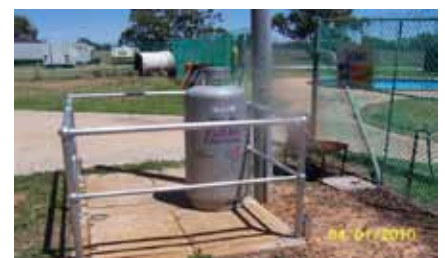
Nagambie Recreation Reserve Kitchen received an upgrade
