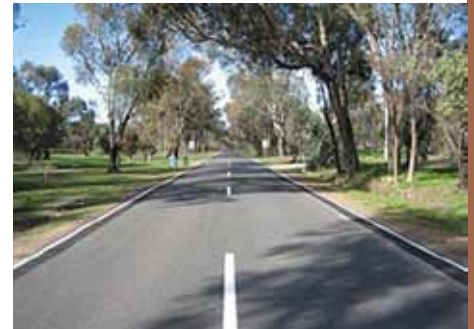
ROAD WIDENING AND WHITE LINE MARKING
