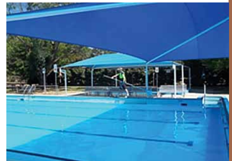
SWIMMING POOL REFURBISHMENT
