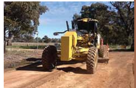
GRAVEL ROAD RE-SHEETING
