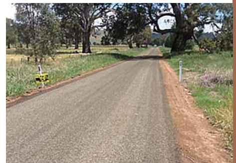
ROAD PAVEMENT REHABILITATION
