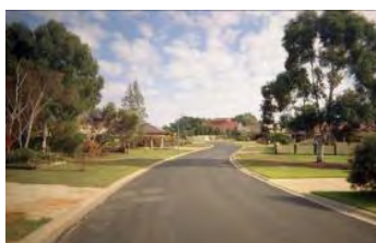
Barwon Street: Needs a footpath.
