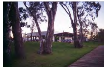
Chinaman’s Bridge Caravan Park Café: A new development that fits in with the natural environment. It allows people to still enjoy the nature around it.
