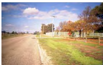
High metal fence in solid colour is a stark contrast to the environment. Looks wrong.
