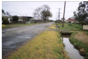
“Open drains and grass verges that... are more in keeping with the rural feel of the township.”
