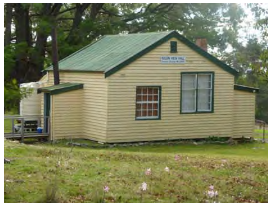
Former School, Kelvin View
