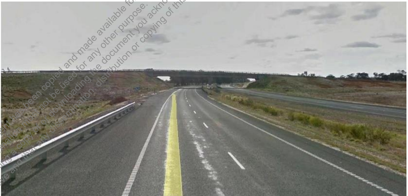
Figure 9: Goulburn Valley Freeway North Direction
