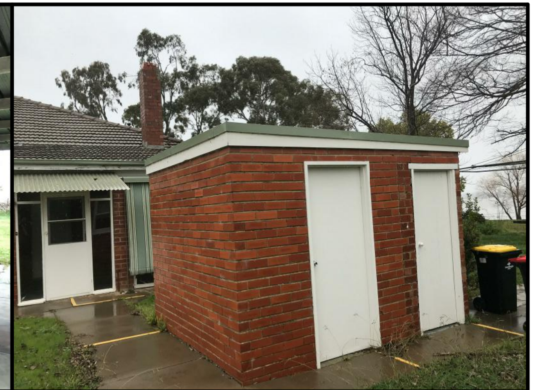
Photograph 8 North East perspective of the existing 2 Bedroom Brick veneer residence & brick toilet block. Existing residence and surrounding sub structures are to be fully demolished as part of the proposed works. Demolish in strict accordance with all relevant standards and regulations. Prepare site for all proposed works
