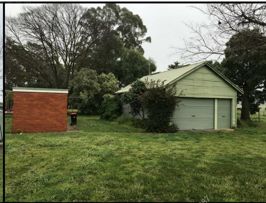
Photograph 3 Eastern perspective of the existing external brick toilet block & rear storage shed/studio. Existing brick toilet block & rear storage shed/studio are to be fully demolished as part of the proposed works. Demolish in strict accordance with all relevant standards and regulations. Prepare site for all proposed works
