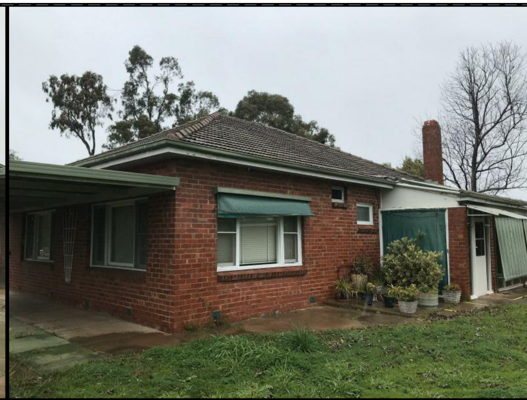
Photograph 2 North East perspective of the existing 2 Bedroom Brick veneer residence. Existing residence and surrounding sub structures are to be fully demolished as part of the proposed works. Demolish in strict accordance with all relevant standards and regulations. Prepare site for all proposed works
