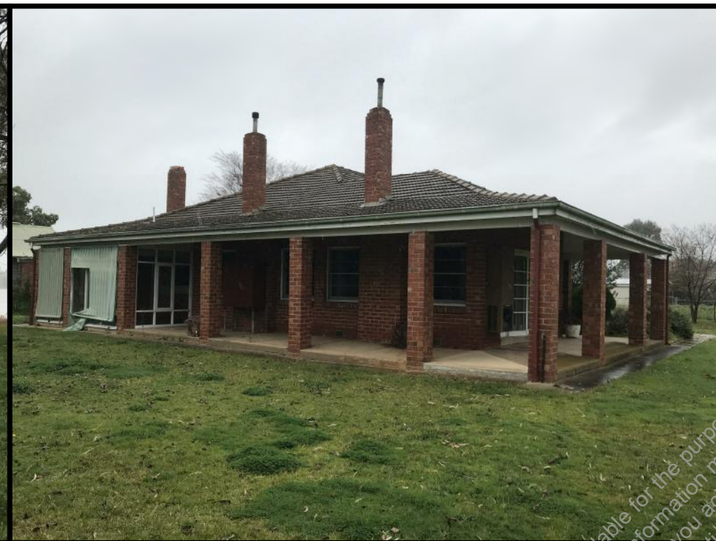
Photograph 6 South West perspective of the existing 2 Bedroom Brick veneer residence. Existing residence and surrounding sub structures are to be fully demolished as part of the proposed works. Demolish in strict accordance with all relevant standards and regulations. Prepare site for all proposed works
