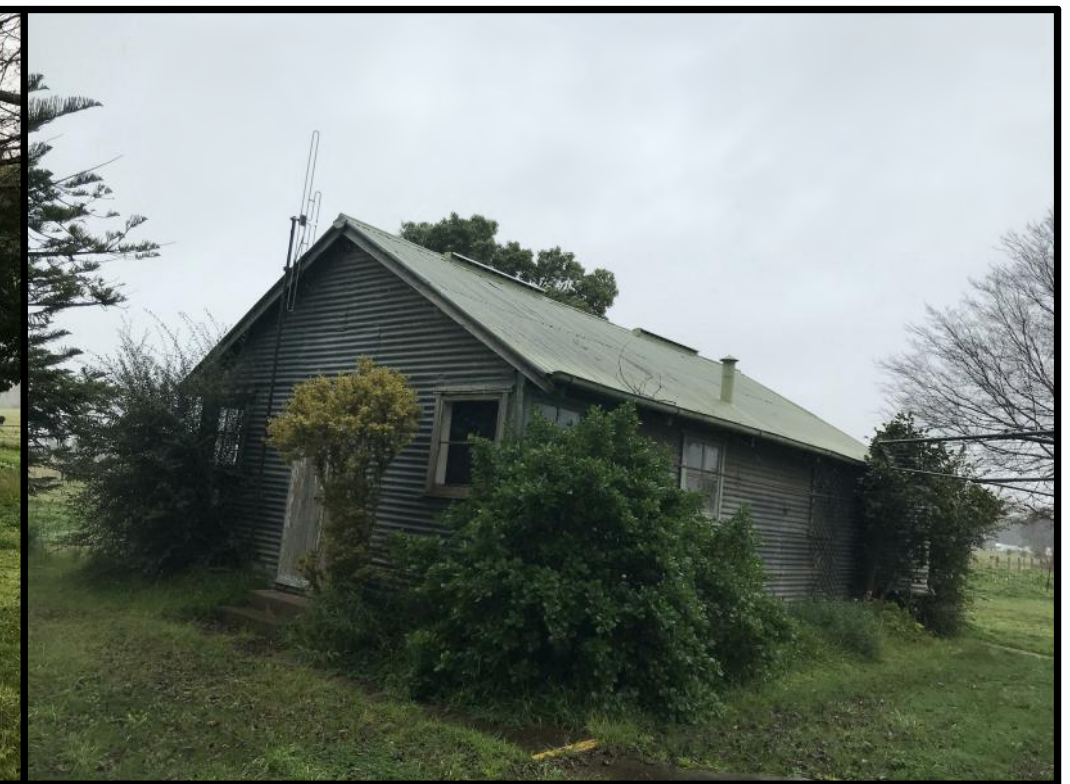
Photograph 4 South West perspective of the existing rear storage shed/studio. Existing rear storage shed & surrounding vegetation are to be fully demolished & removed as part of the proposed works. Demolish in strict accordance with all relevant standards and regulations. Prepare site for all proposed works
