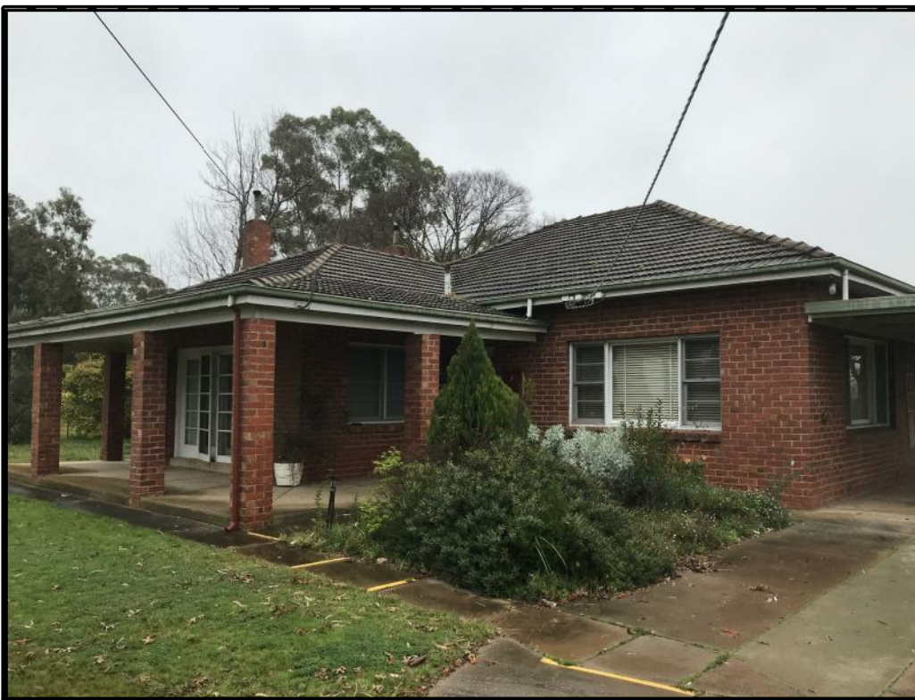
Photograph 1 South East perspective of the existing 2 Bedroom Brick veneer residence. Existing residence and surrounding sub structures are to be fully demolished as part of the proposed works. Demolish in strict accordance with all relevant standards and regulations. Remove vegetation shown to the front of the existing residence. Prepare site for all proposed works
