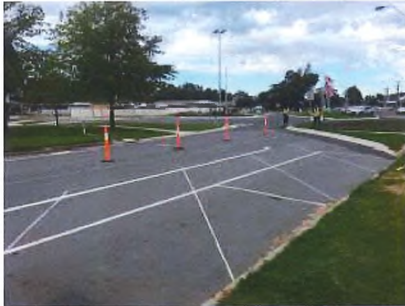
Photo 1: Easement layout with reversing area. Edge of bollards represents edge of the through traffic lane
