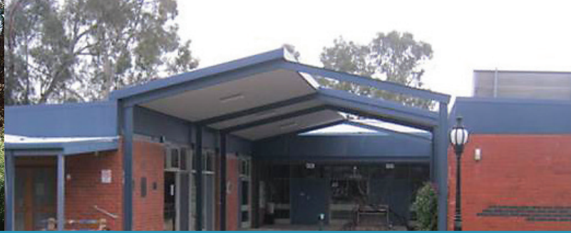
Violet Town Community Complex re-roofed
