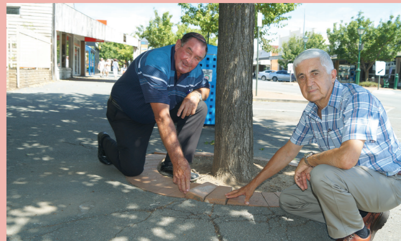
Seven Creeks Ward Councillors Mick Williams and John Mason inspect the damage caused by invasive tree roots on Binney Street.
