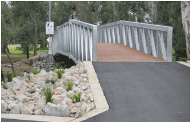
The Euroa Caravan Park Restoration.
