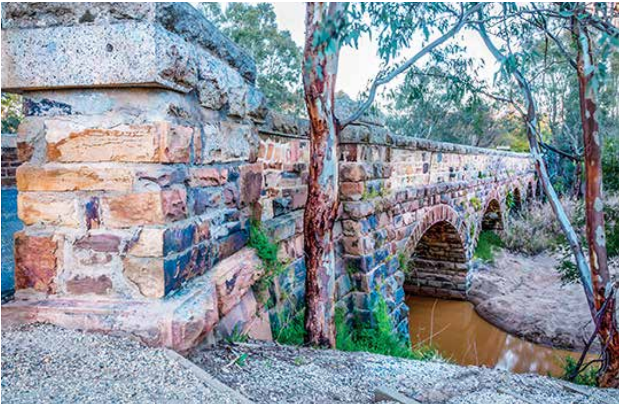
Historical Avenel Bridge over Hughes Creek, Avenel
