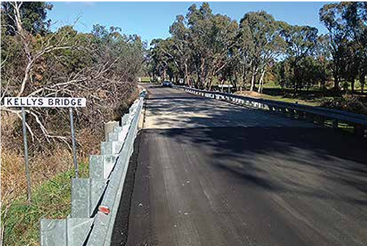
Kellys Bridge - re-deck, Creightons Creek
