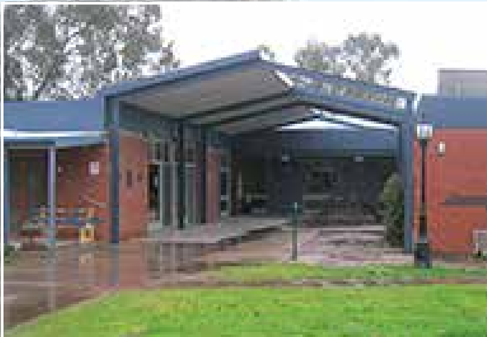
Violet Town Community Centre ~ new roofing
